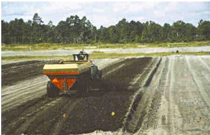
A standard agricultural manure spreader can be used to apply compost blankets on minor slopes.
